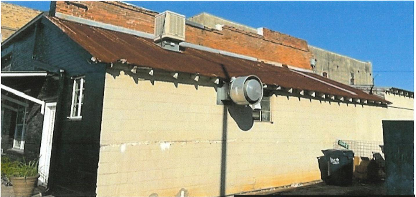
Replace Rusted Roofing and repair Wooden rafters and supports as needed. New roofing will match the metal roofing on the rest of the building. This roofing suffers from wear and trucks hitting it over the years. The large square box on the roof is not used and will be removed and not replaced.
